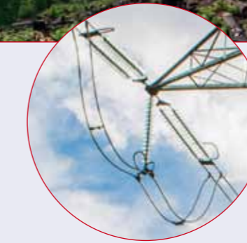
Special suspension clamps for conductor and ground wire installed on a long river crossing span (about 2 km) in Nigeria
