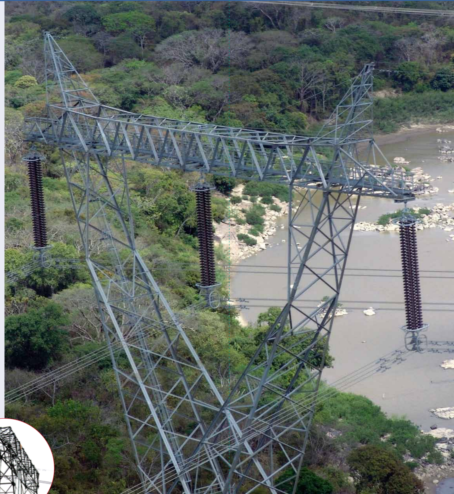
Special suspension clamps for conductor and ground wire installed on a long river crossing span (about 2 km) in Nigeria
